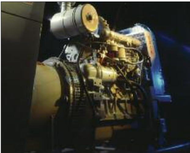
Diesel Generator Set. Coupling fitted between the engine and alternator.
